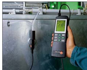
Measuring differential pressure when changing a filter
